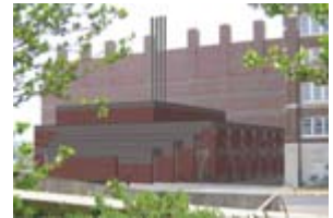
Construction on the first building at UT-Baptist Research Park, the Regional Biocontainment Laboratory (pictured above), is expected to be complete in 2008.
